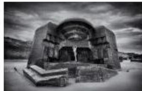
Broken bunker 5006MCT
